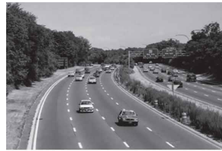
(a) A Typical 8-Lane Freeway
